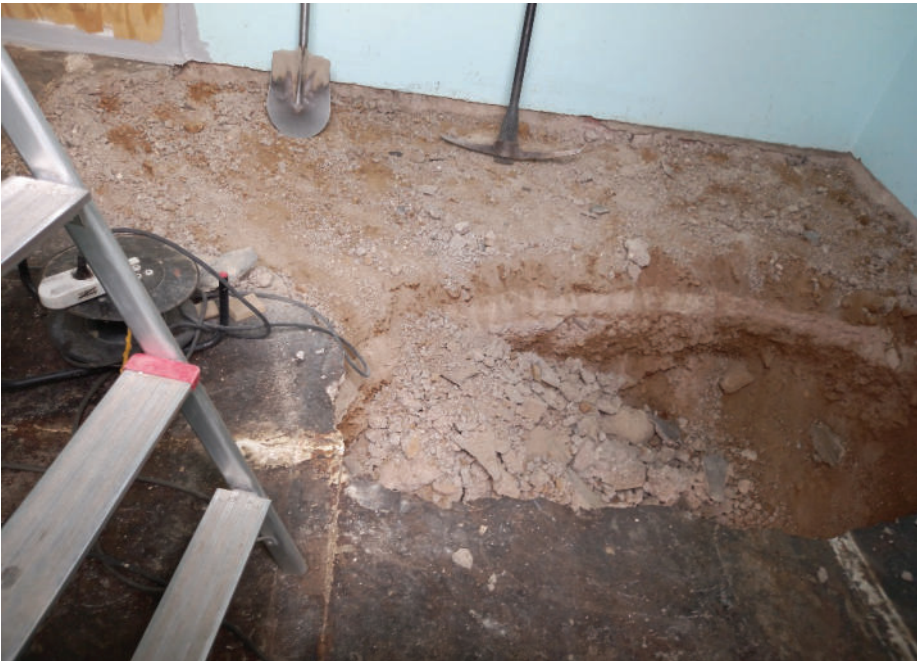
Digging deeper and deeper
