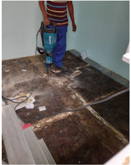
The work begins
