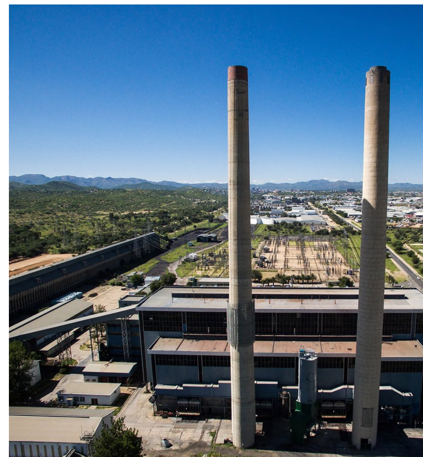
Source: Hans Rack - Van Eck power station
