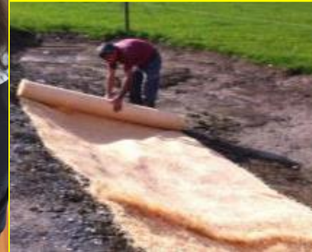
Wood-wool erosion blankets & bio-char
